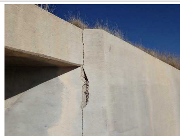
Cracking and spalling at CBC/Wingwall joint of Bridge No. 9438
