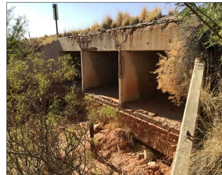
NM 31 3-Barrel CBC: Milepost 11.88, Bridge No. 7976
